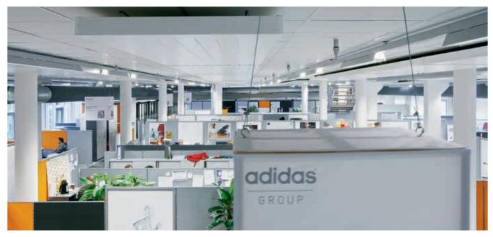
Areas where warm air collects in larger quantities must receive more cooling – and vice-versa. Thanks to the high radiation component of the flat panels, a comfortable indoor climate is achieved with high efficiency.
