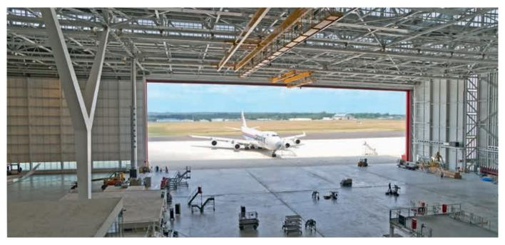
17,000 m<sup>2</sup> floor space, and a ceiling height of up to 42 m: an enormous challenge for Versatile ZBN. The principle of thermal radiation takes full effect here, particularly considering that the heat is required mainly in the lower area of the hall.
