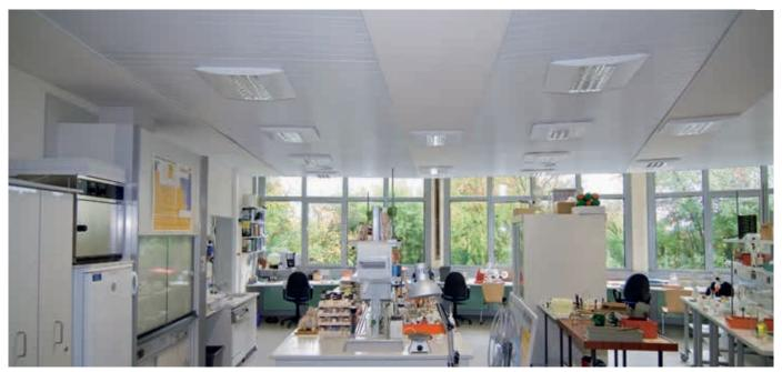
And the result was a lesson to all: the system was also installed in the chemistry area, in combination with a ventilation system. Inlets and outlets were integrated flush in the ceiling sails; the lighting was fitted on the sails.
