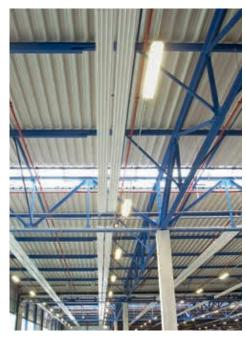
Emphasis is also placed on performance and efficiency in the area of climate-control technology, in the form of a Versatile radiant ceiling system. 19km of Versatile ZIP radiant panels were installed.
