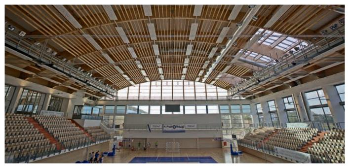
In order to heat the 5000 m<sup>2</sup> large hall evenly and efficiently, the decision was made to choose Versatile ZBN. A total of 372 m<sup>2</sup> of perforated radiant panels for noise reduction were installed on the wooden structure which supports the roof of the hall.
