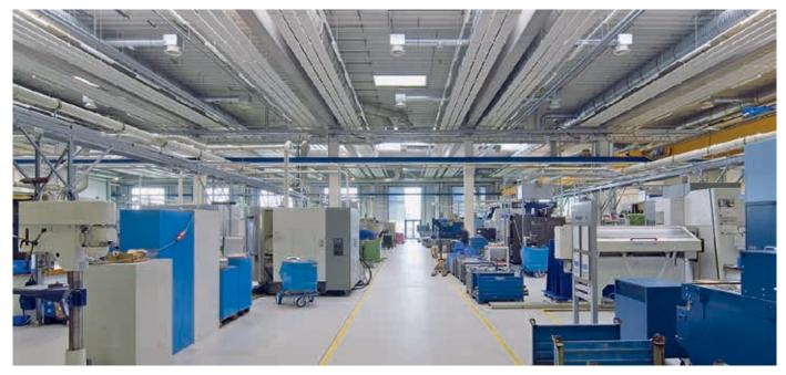
Versatile ZIP or Versatile Como products were utilised, depending on the individual department and its particular requirements. Ventilation outlets and lighting elements were integrated into the enclosed Versatile Como ceiling sails.
