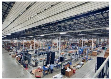
Versatile ZIP radiant panels were used. An overall length of approximately 1800 m was installed in 13,000 m<sup>2</sup> of plant area and 1850 m<sup>2</sup> of office space, with ceilings ranging up to 30 m in height.
