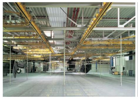
A total of 419 Versatile radiant ceiling panel elements were installed in the new assembly halls. Their suspension was integrated without difficulty in the complex production lines of the fully automated paint shop.
