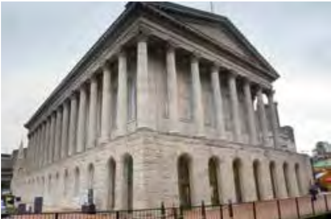
Birmingham Town Hall - Clima Canal
