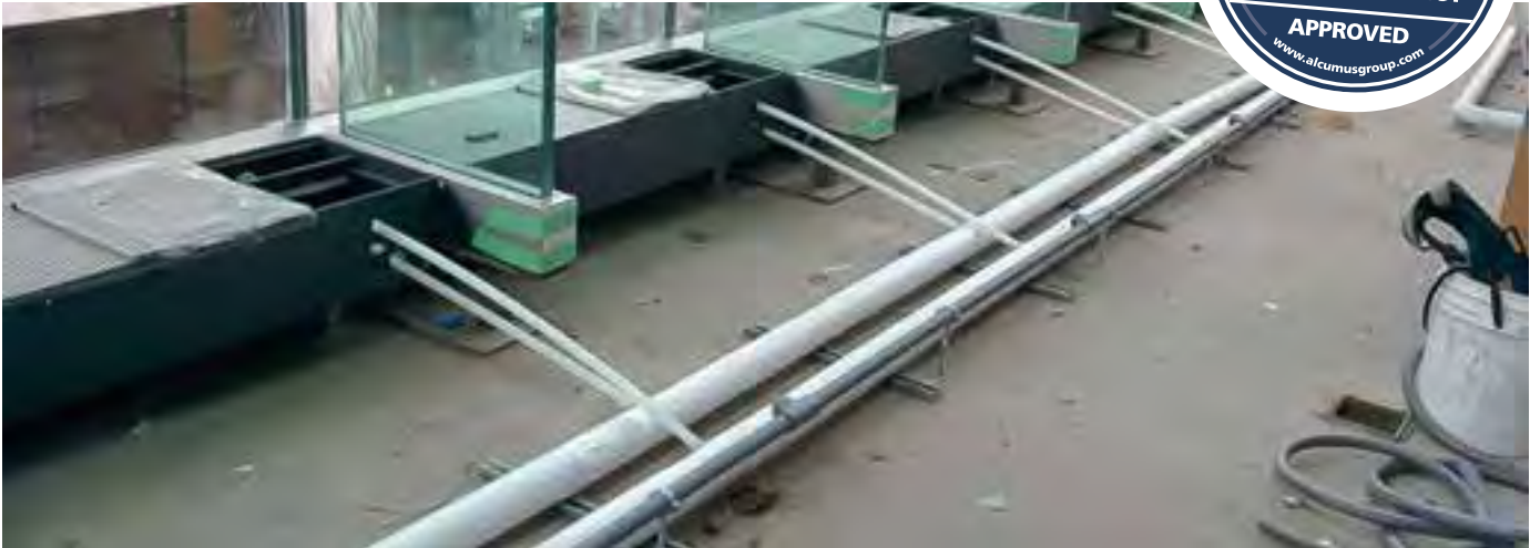
Clima Canal: Installation
