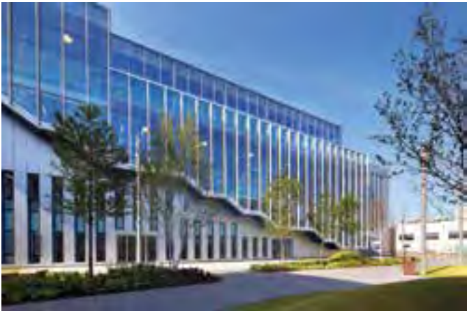
Sky Believe in Better Building - Mini Canal (BREEAM Excellent)
