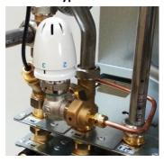
The "Summer bypass" valve utilises a return temperature limiter head fitted to a thermostatic valve installed in a bypass between the primary flow and return pipework within the HIU. This maintains a minimum primary temperature when the space heating is not in use.
